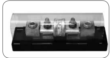
Fig. 3.15. Class "T" Fuse Assembly
